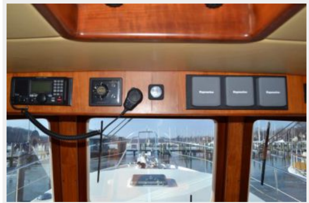
49' Krogen Express pilothouse overhead electronics
