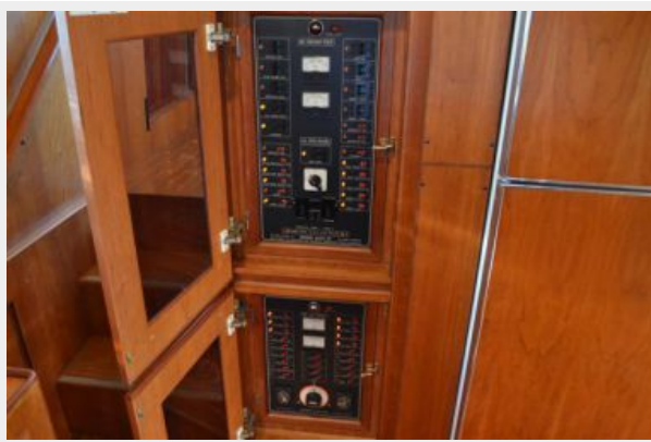
49' Krogen Express electrical panel
