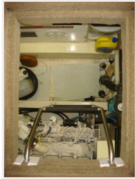
34' American Tug engine room access
