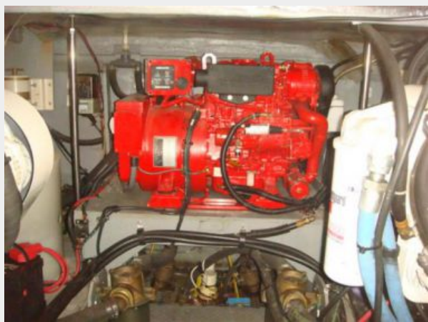
45' Sea Ray engine room forward
