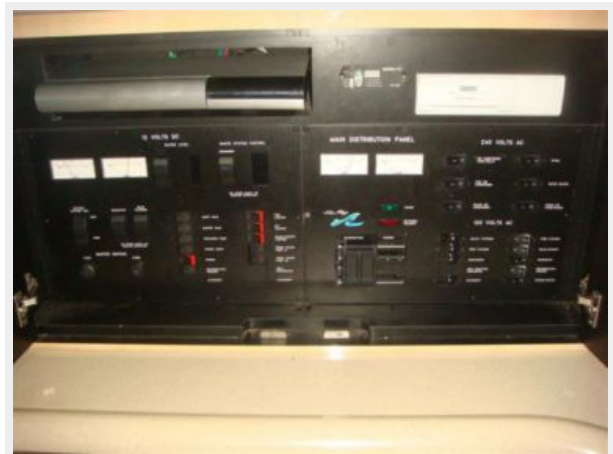
45' Sea Ray electrical panel
