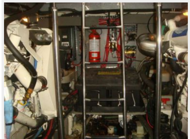
45' Sea Ray engine room aft
