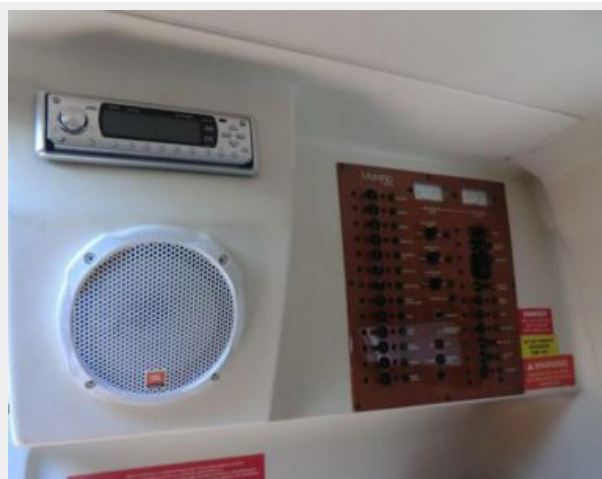
Electrical Panel and Stereo
