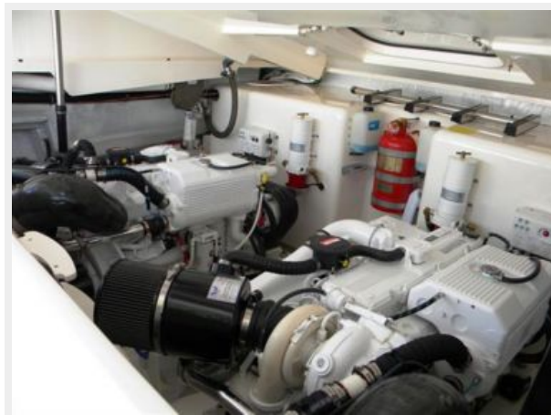
Engine Room Starboard
