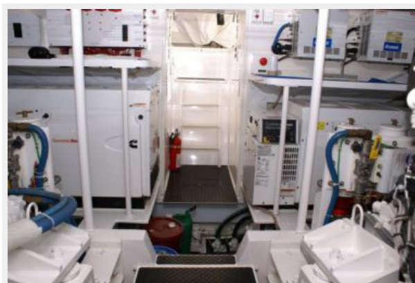
Engine Room Entry & Generators
