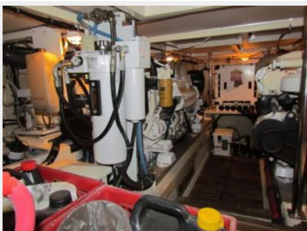
Enginr Room Starboard
