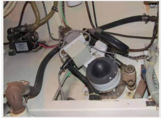
Engine Room Port Stabilizer
