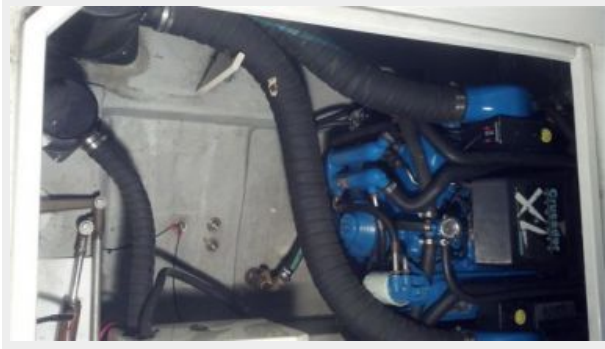
Port eng after replacement, 8-20-14
