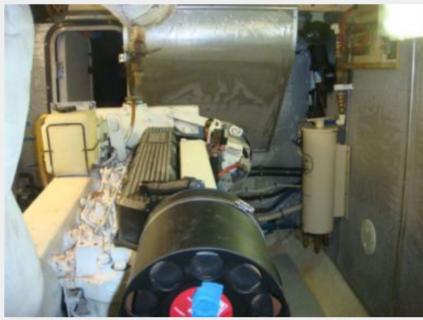
40' Nordhavn engine room forward
