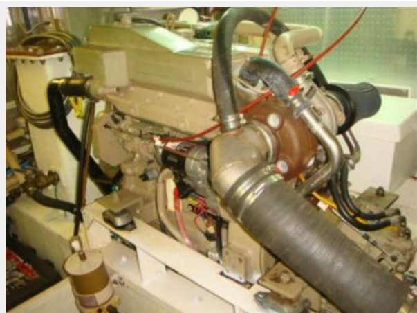
49' DeFever starboard main engine photo2
