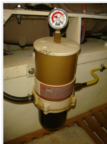
49' DeFever starboard Racor fuel filter
