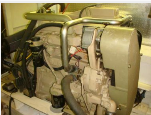
49' DeFever port main engine photo1
