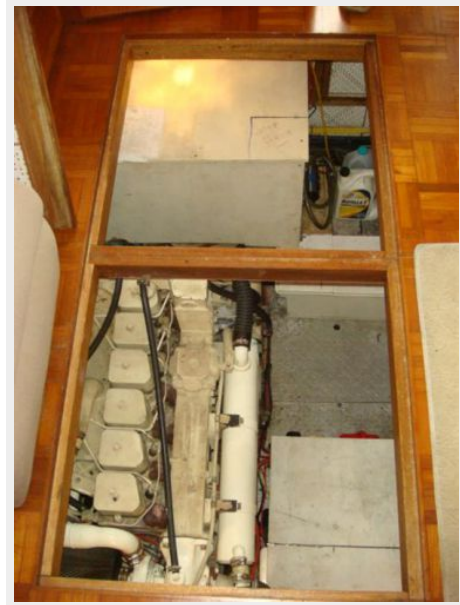
42' Jefferson engine room access
