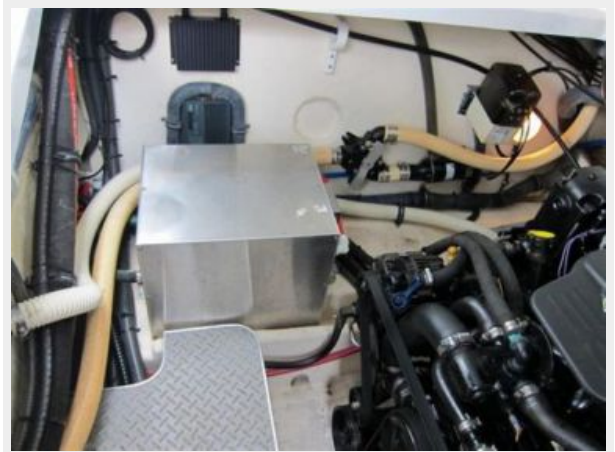
Spotless Engine room
