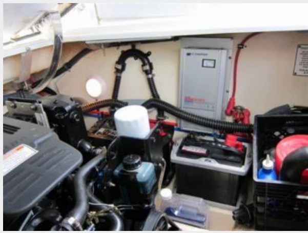
Spotless Engine room
