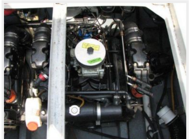
Engine & Mechanical Equipment 1 - Port Engine
