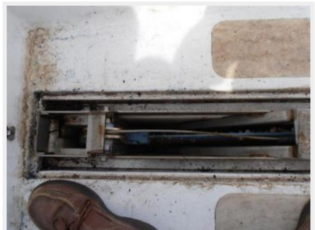
Cap removed on the lead keel
