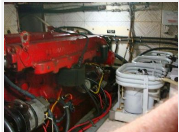
41' DeFever engine room port aft
