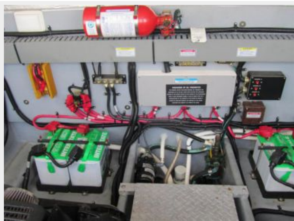
33' Sea Ray engine room forward
