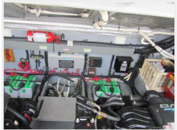
33' Sea Ray engine room
