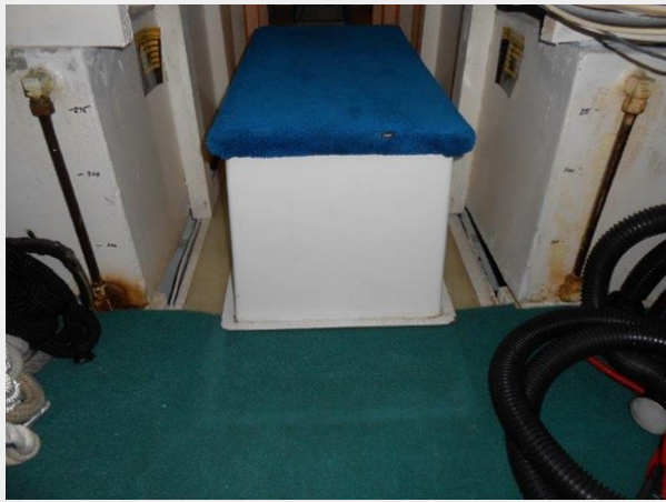
Lazarette Fuel Tanks
