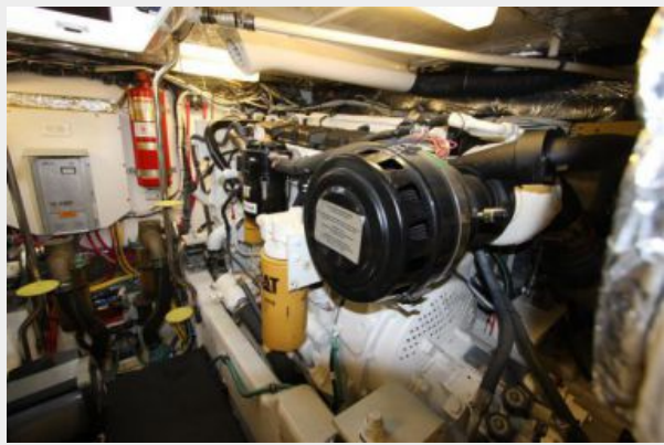
Engine Room Starboard Forward
