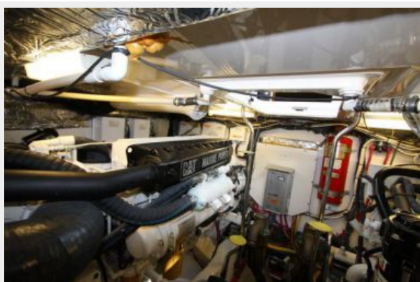
Engine Room Forward
