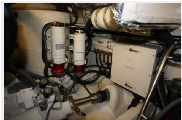
Engine Room/Racor Fuel Filters
