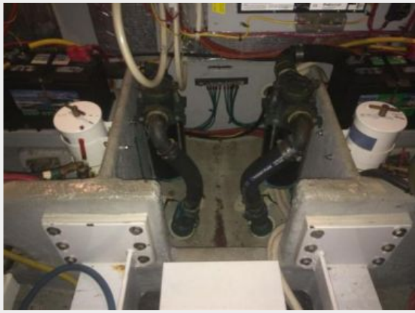
Engine Room - Facing Aft
