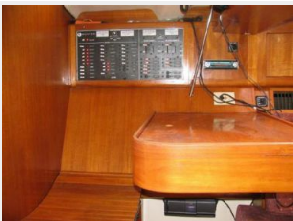
AC and DC electrical panel
