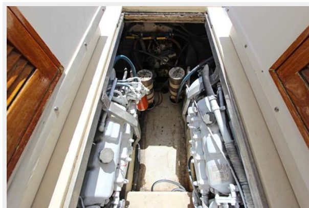
Engine Room Access Between Helm Seating
