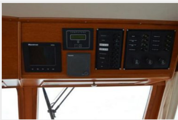
Lower Helm Electronics & Panel
