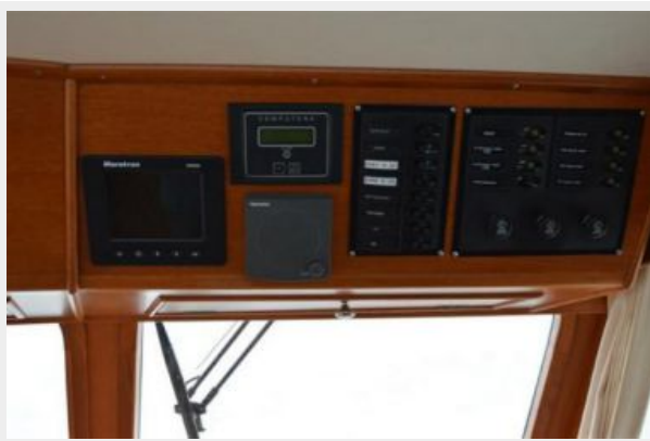
Lower Helm Electronics & Panel
