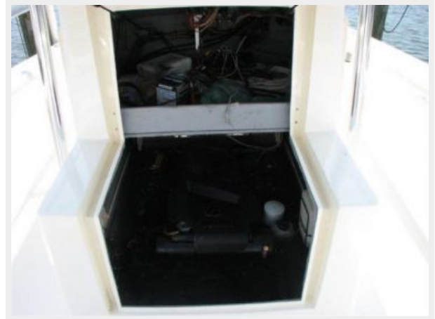
Engine & Mechanical Equipment 1 - Engine Room
