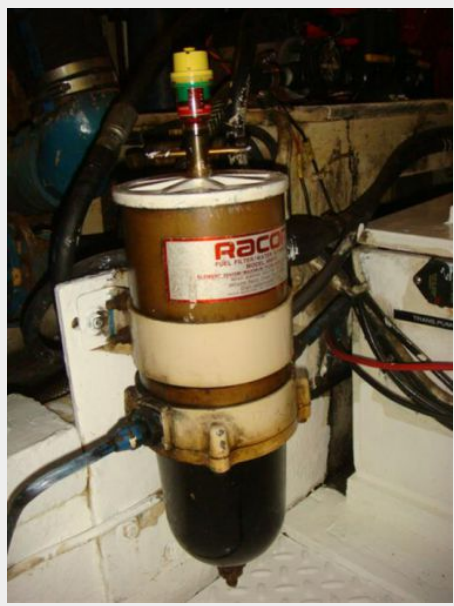
44' DeFever port Racor fuel filter
