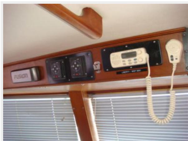
44' DeFever lower helm overhead electronics photo2
