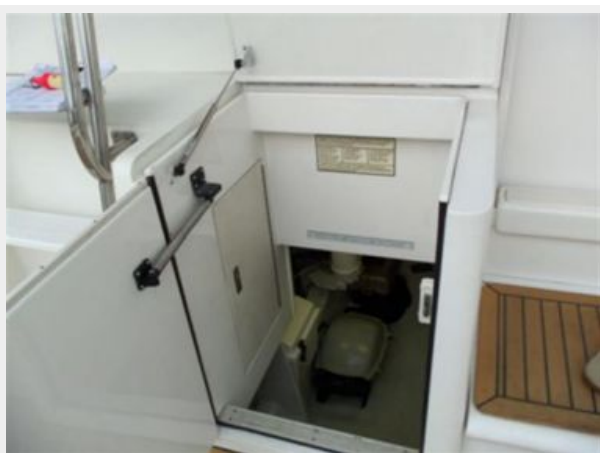
Engine room access
