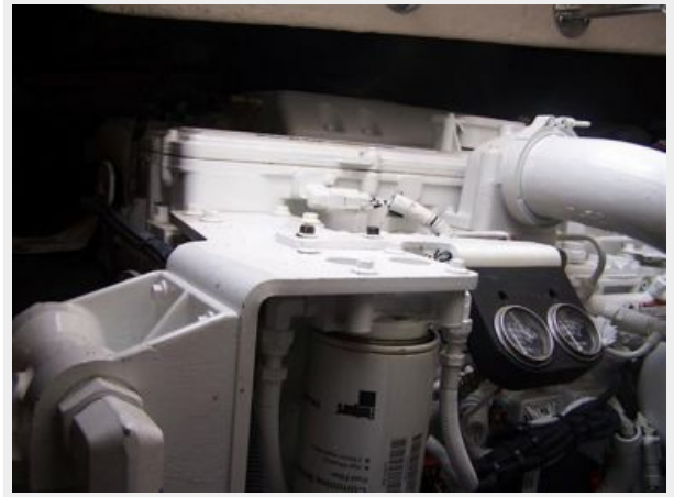
Engine Room Equipment
