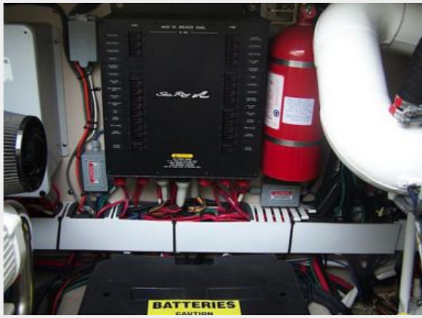
Engine Room Equipment
