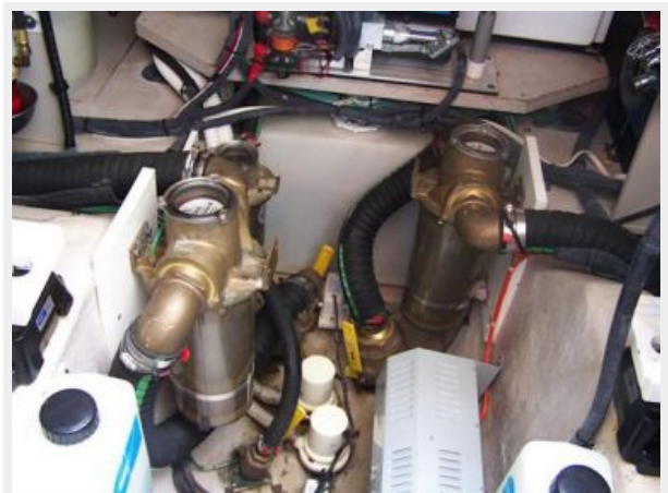
Strainers and Bilge Heater
