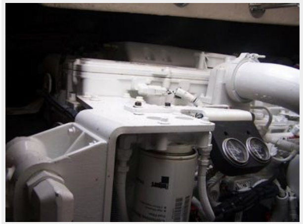
Engine Room Equipment
