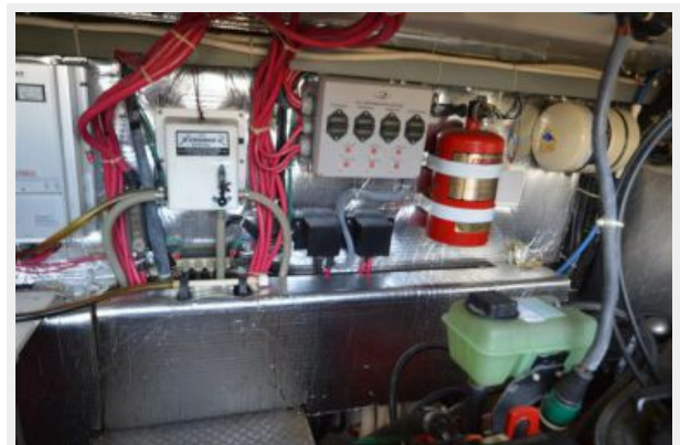
'03 Regal 3860; Fire Suppression System
