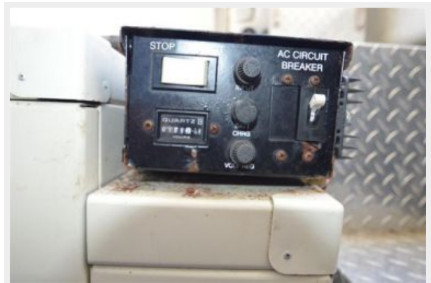
'03 Regal 3860; Generator Hours
