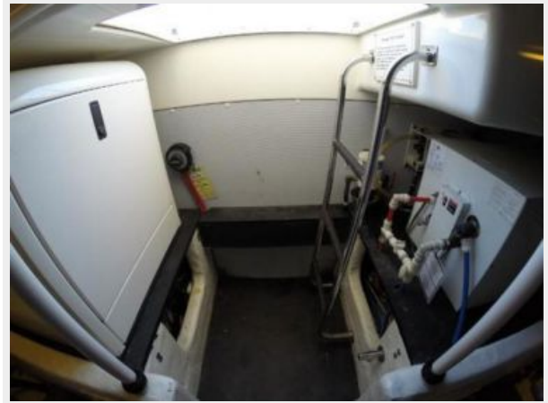
Engine Room (facing Aft)
