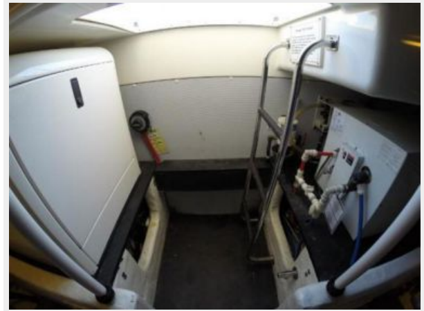
Engine Room (facing Aft)
