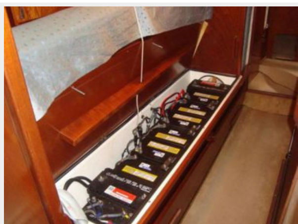
Battery Storage - Sea Berth
