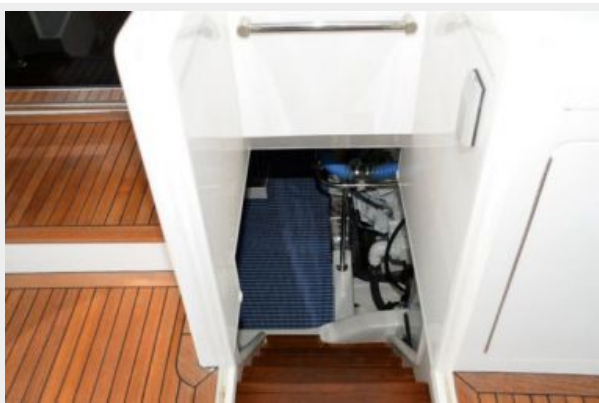
Walk-in Engine Room Access
