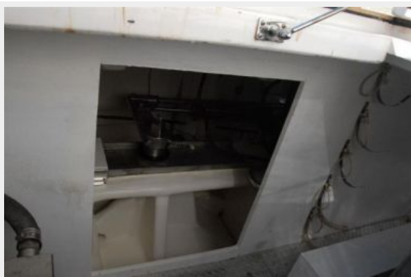
Rudder Access from Lazarette
