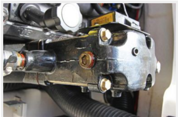
New Risers/Manifolds September 2013
