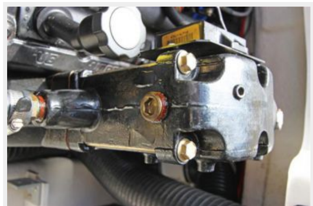
New Risers/Manifolds September 2013
