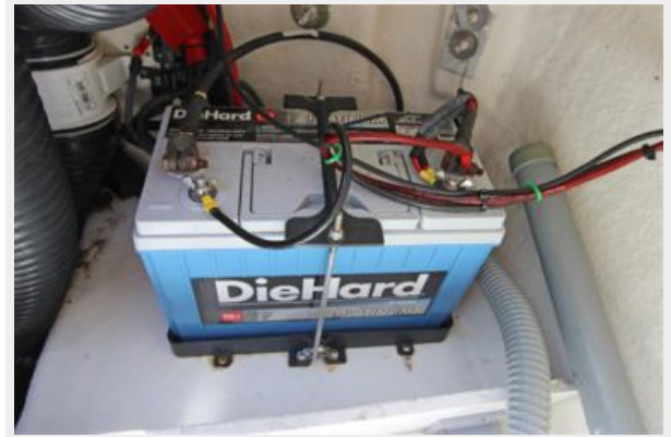
Battery Mounted In Tray
