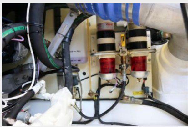
Engine Room Dual Racor Filters
