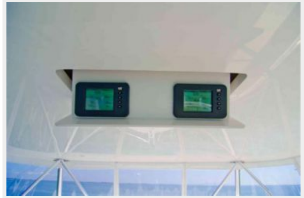
Flybridge Helm Electronics
