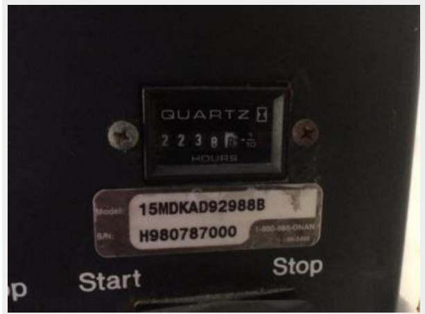
15 kW Onan Generator with 2238 hours
