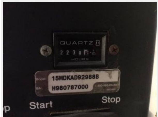
15 kW Onan Generator with 2238 hours
