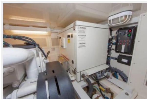
Engine Room Port Forward with Generator
