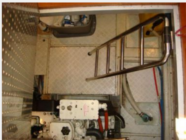
37' Mariner Seville engine room forward access
