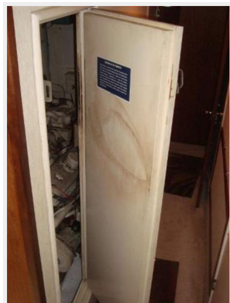
Engine room access
