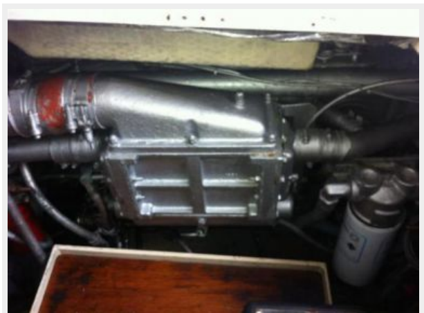
Engine room (port)
