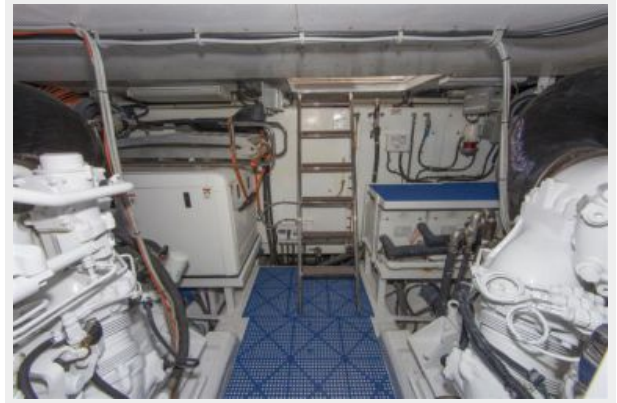
Engine Room Looking Aft
