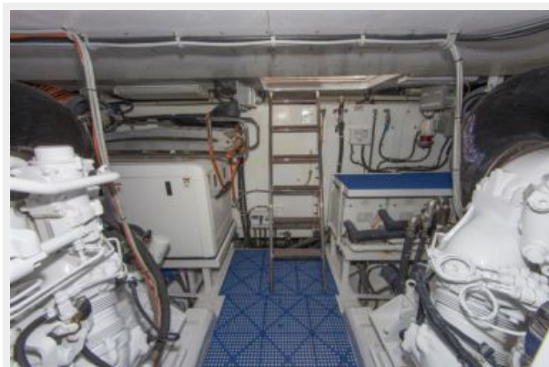
Engine Room Looking Aft
