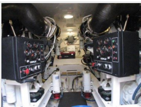
Engine & Mechanical Equipment 1 - Engine Room
